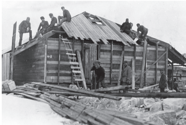
Building Mawson's Hut in 1912. Frank Hurley photo.
